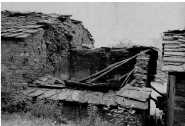
Fig. 13: Roof Collapse due to lack of Anchorage
