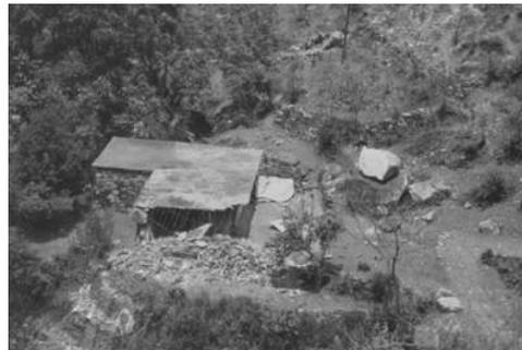
Fig. 8 : Building Damage due to rockfall
